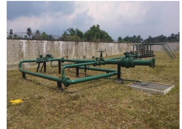
Oza Manifold & Pipeline Launcher
