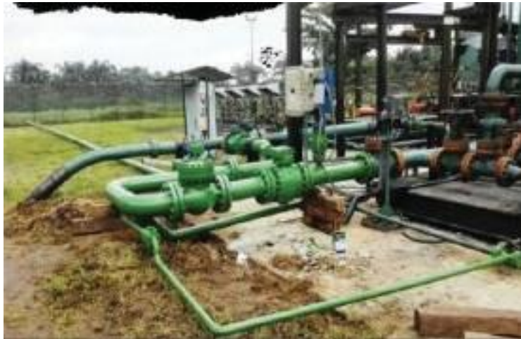
Tie-in Point to Trans Niger Pipeline
